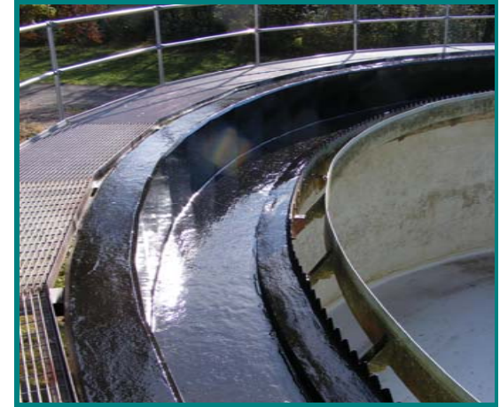
Completed silicone fouling release system ready for immersion service
