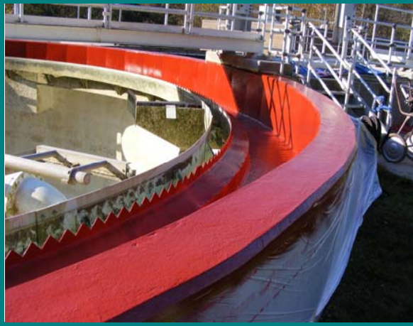
Second coat of epoxy
