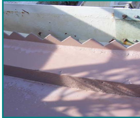
Silicone Tie Coat ready for application of silicone Surface Coat
