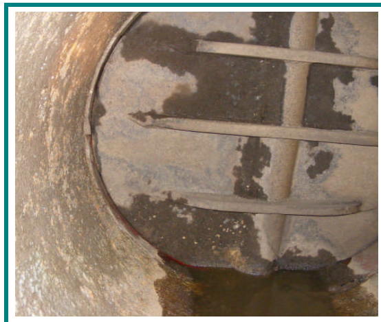
Tunnel #11, control gate, March 9, 2008
